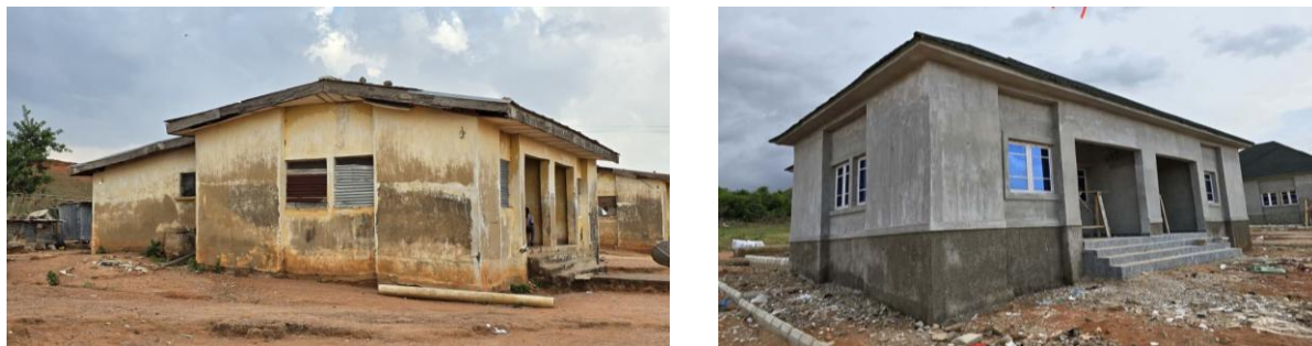
Plate 1: Old and renovated 'C' block of MKCB, Bassa LGA with louvre window and newly installed casement window respectively.
