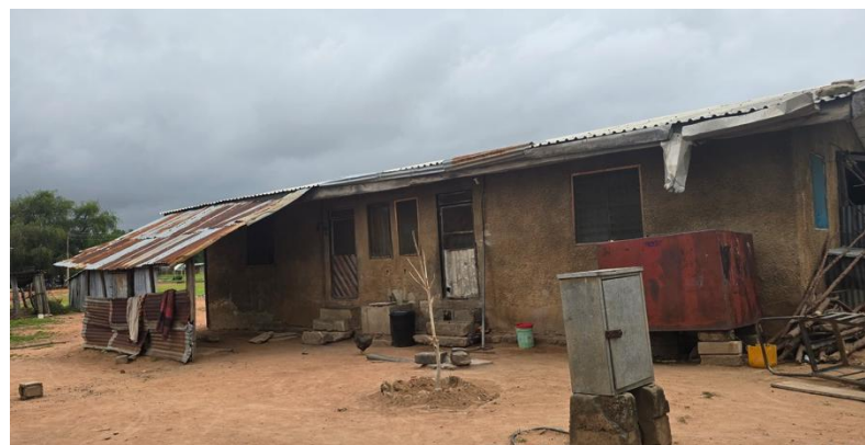
Plate 2: 'C' block ARB, Shendam with louvre windows.
